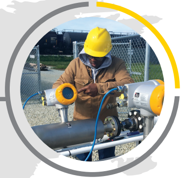
Customer Support On-Site Commissioning
